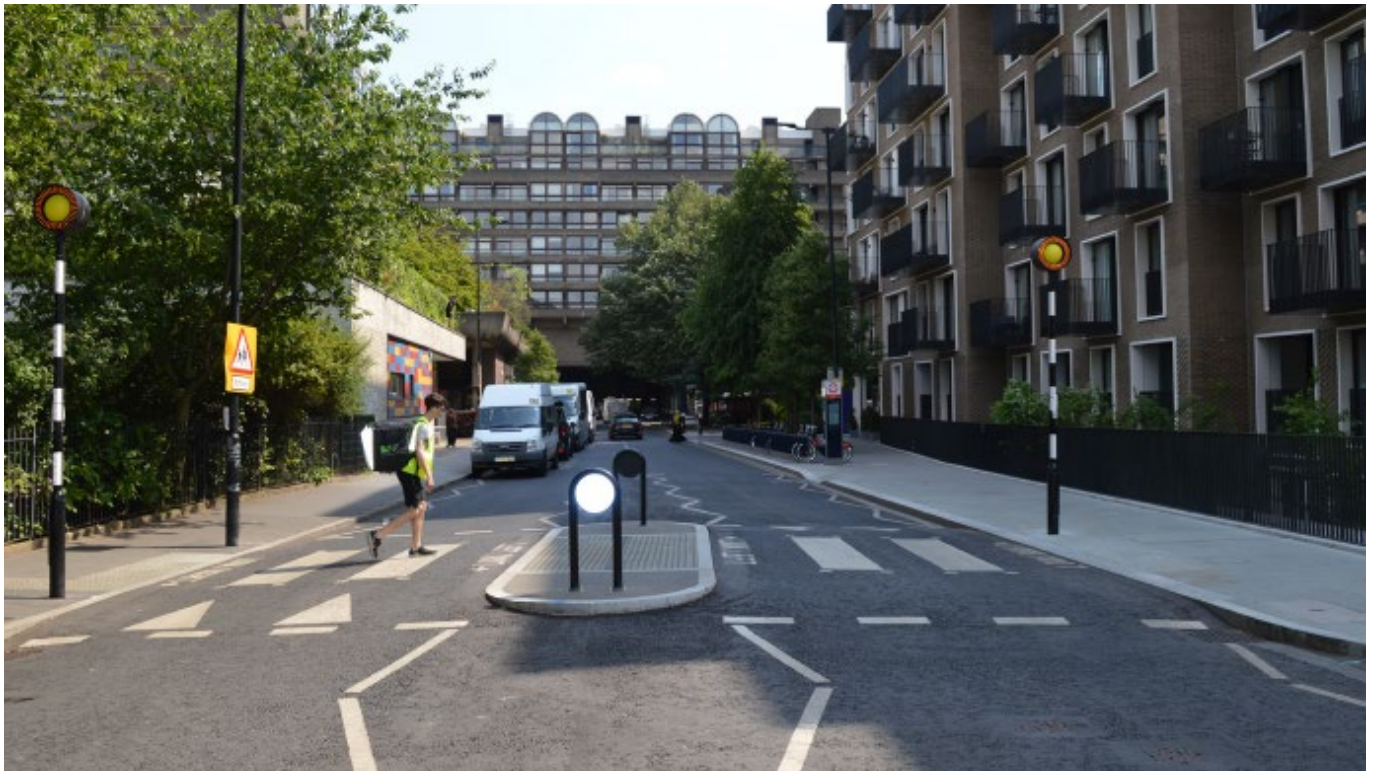
Figure 1211: A newly completed raised zebra crossing on Golden Lane.
