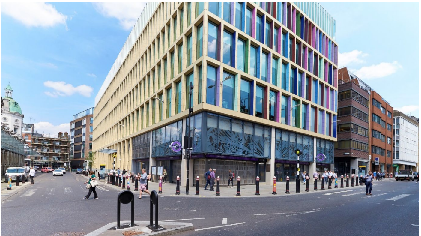
Figure 2220: The entrance to the new Farringdon entrance to the Elizabeth line on the Corner of Long Lane and Lindsey Street. ©Clive Totman
